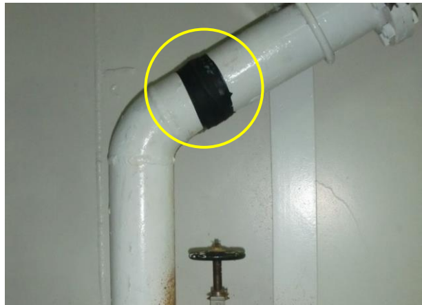
Pipe temporarily repaired with rubber patch.
