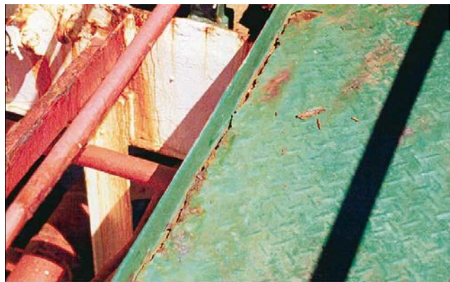
Catwalk cracked.
