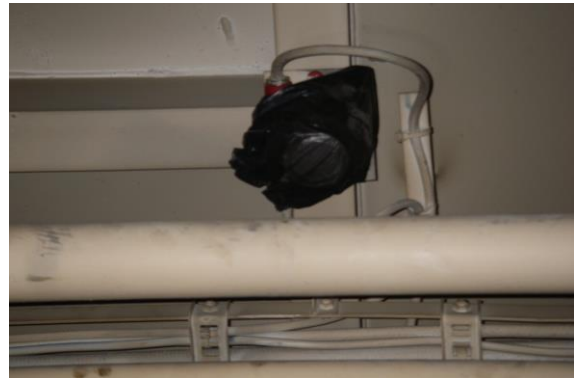
Smoke detector covered by plastic bag.
